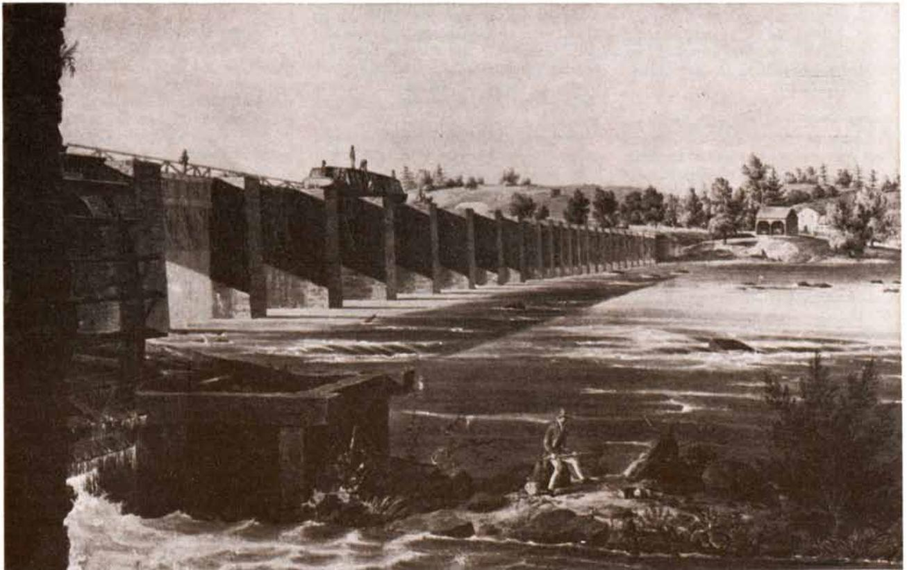
**CANAL AQUEDUCTS ON THE ERIE** enabled the barges to cross streams encountered along the right-of-way. This painting by Hill
