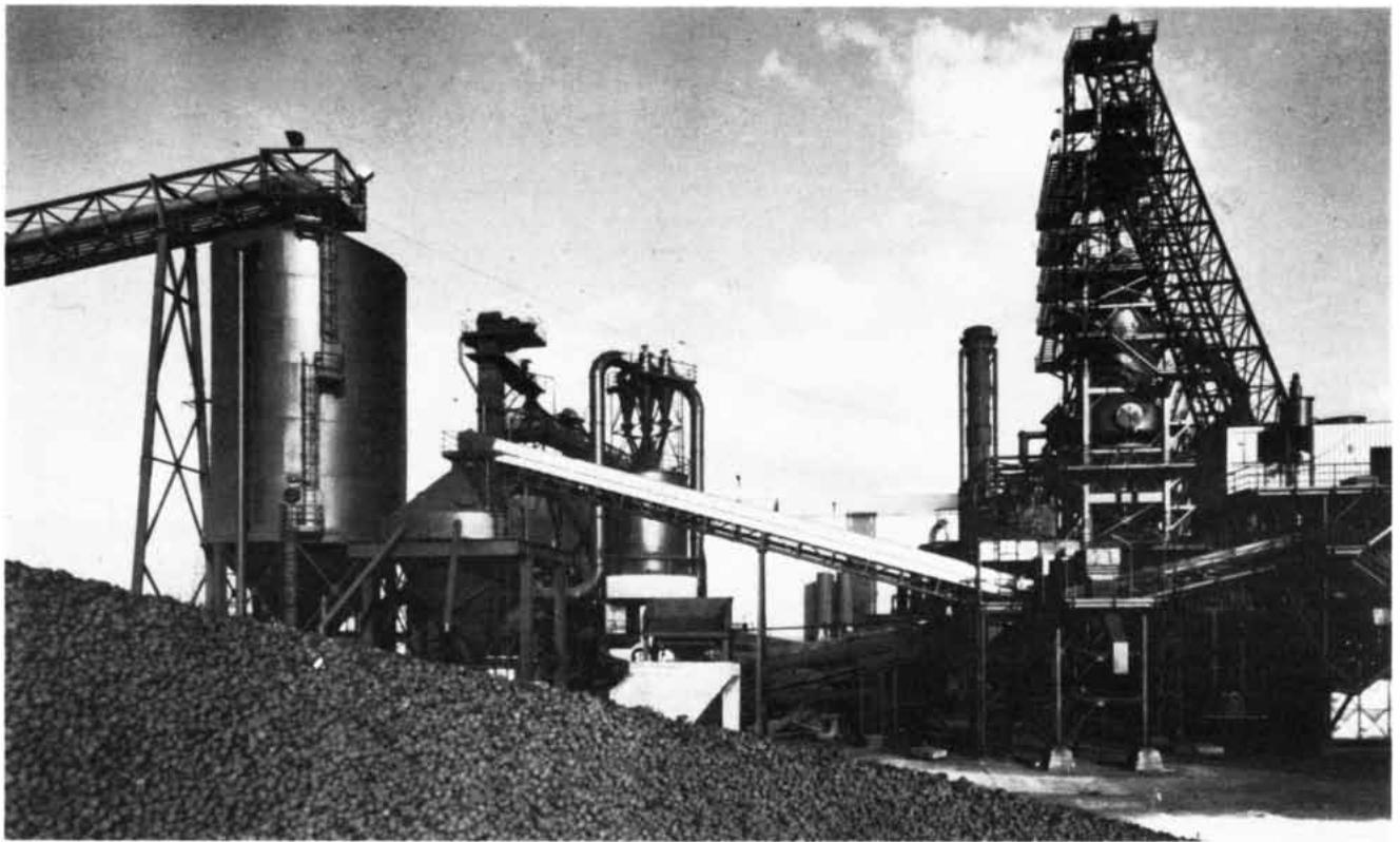
**MIDREX PLANT** is operated in Hamburg, West Germany, by Korf Industries, Inc. It has a capacity of 350,000 tons of sponge iron per year. At right is the reducing stack, which has a skip-car charging system. The tall silo at left is a "day bin" in which iron ore and pellets are stored before being transferred by the dark conveyor at center
