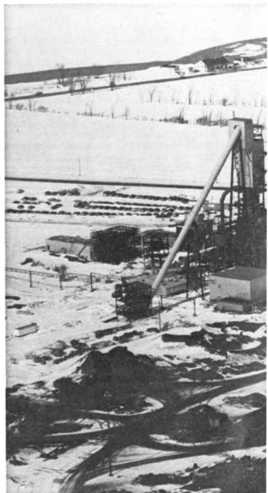
**DIRECT-REDUCTION PLANT** is operated by Sidbec at Contrecoeur in the Canadian province of Quebec. It consists of two modules, each of which is identifiable by a tall shaft with a charging conveyor that runs from the ground to the top of the shaft. The module
