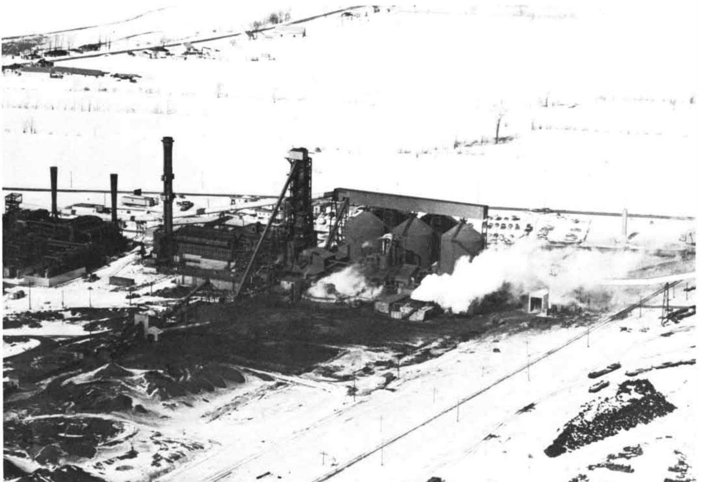
at the right has been in operation since 1973, producing 400,000 tons of directly reduced iron per year. The module at the left is under construction; its capacity will be 650,000 tons per year. The plant employs the Midrex direct-reduction process, in which a charge of lumps of iron ore and pellets of iron oxide is loaded into the shaft through the conveyor and then descends through a stream of hot reducing gas.
