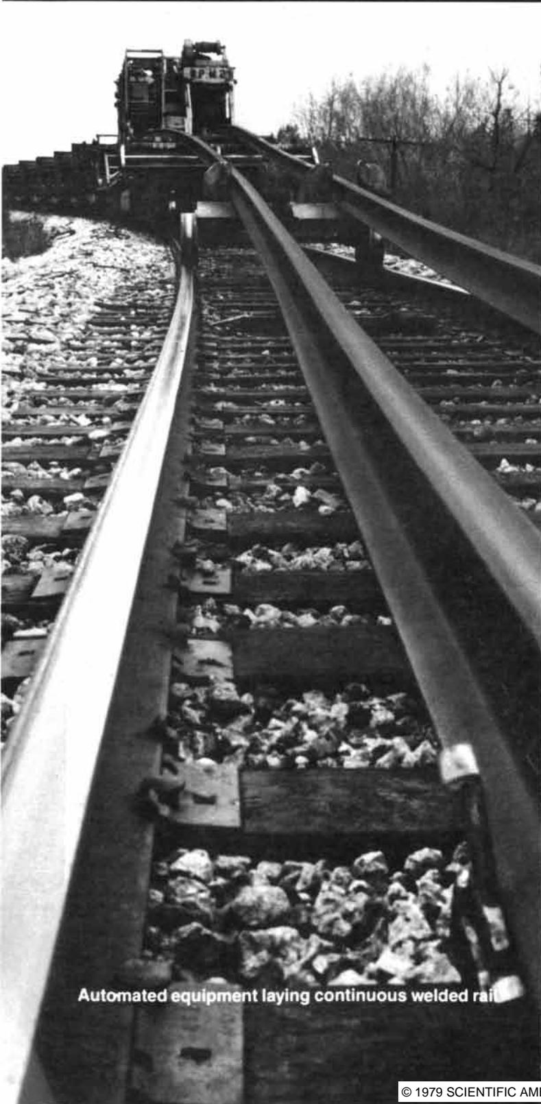
Automated equipment laying continuous welded rail
