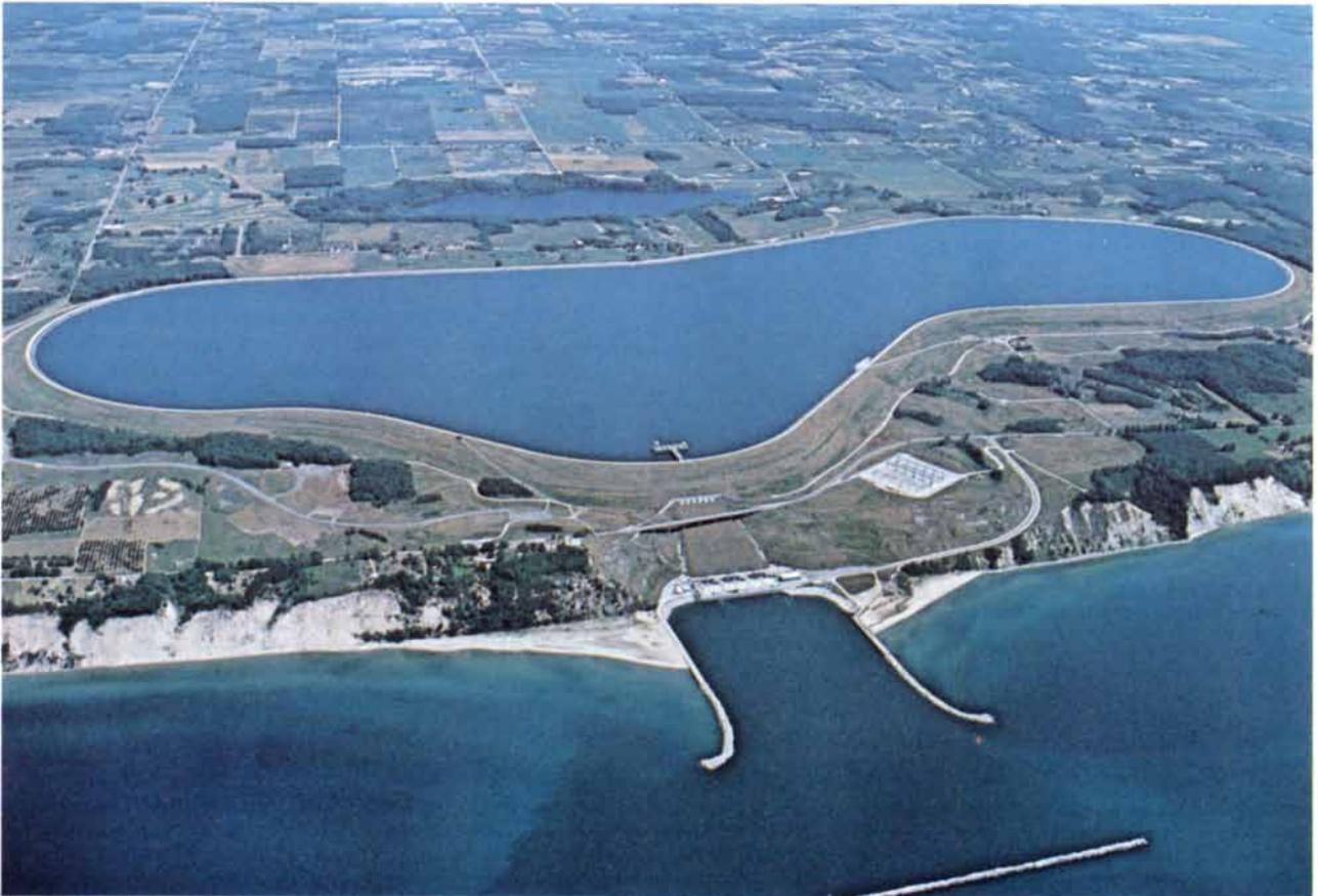
**PUMPED-STORAGE HYDROELECTRIC PLANT** at Ludington on the eastern shore of Lake Michigan is the largest electric-energy storage facility in the world. Off-peak power, available primarily at night and on weekends, is fed to six pump-turbines that raise the water an average of 250 feet from the lower reservoir, Lake Michigan, to the upper reservoir, an artificial lake contained by an earth-fill dam six miles long. At hours of peak electric demand the water in
